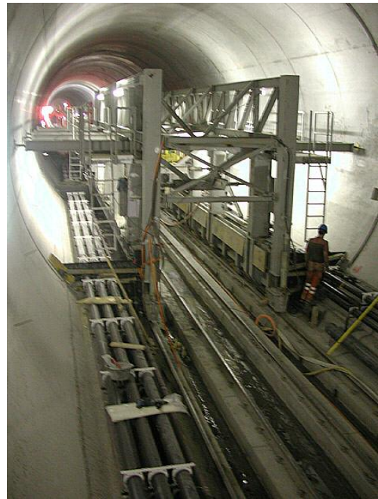
The formwork platform in the Lötschberg tunnel; at the bottom on the left and on the right side of the rails, the conduit blocks ready to concrete-cast.
