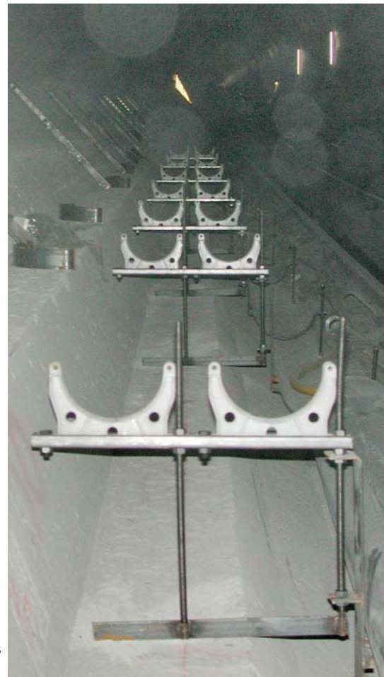
The formwork platform in the Lötschberg tunnel; at the bottom on the left and on the right side of the rails, the conduit blocks ready to concrete-cast.
